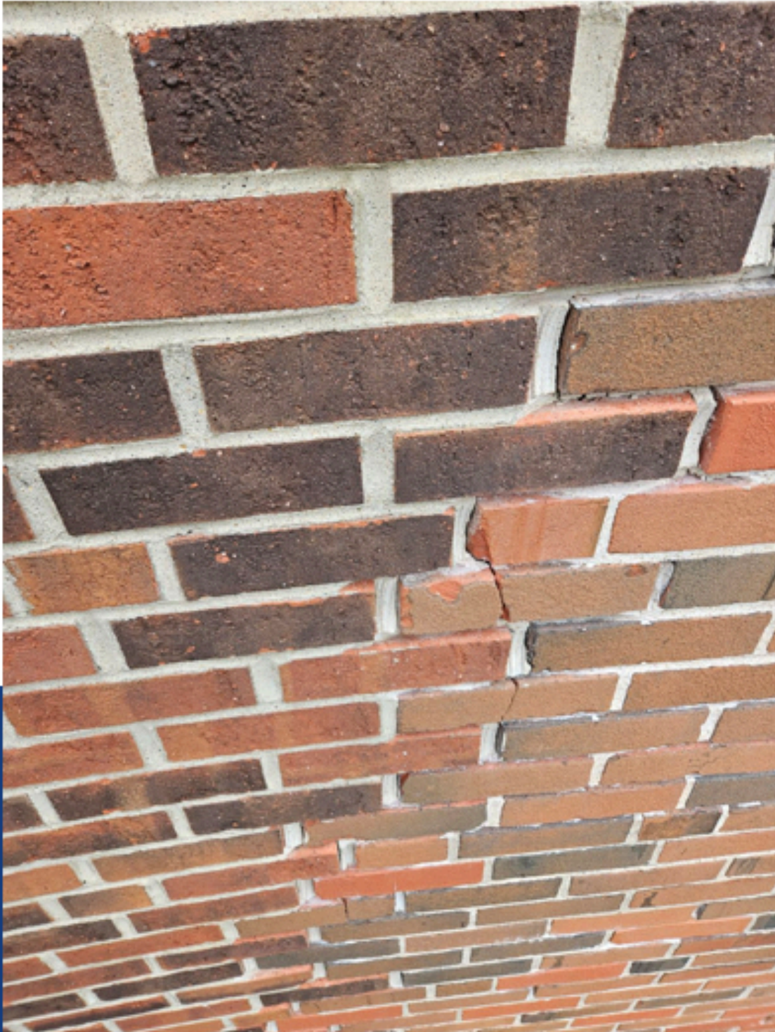
BEFORE - Masonry Repair
